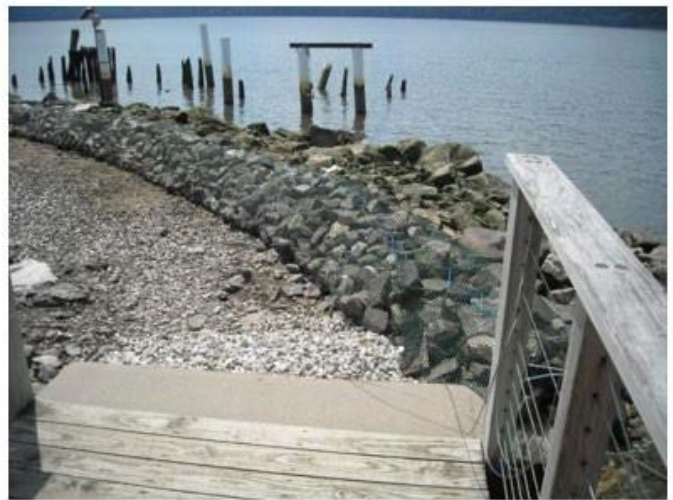
Figure 4: Additional rock added to the sill in 2008 to prevent erosions and control driftwood
