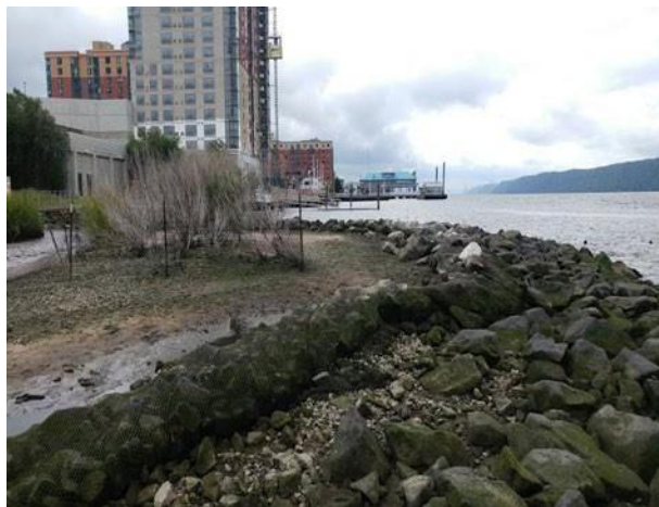
Figure C and D: Left photo looking south at sill, right photo looking east from water at sill and footbridge. Additional rock was installed in 2005 and 2007 to raise the height of the sill. The top layer of rip-rap was enclosed in netting to hold it in place. (Photo taken 9/2018).
