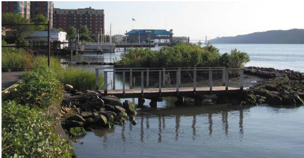
Figure 2: Completed shoreline stabilization and footbridge, September 2012.
