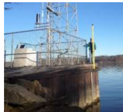
Water Level Station
